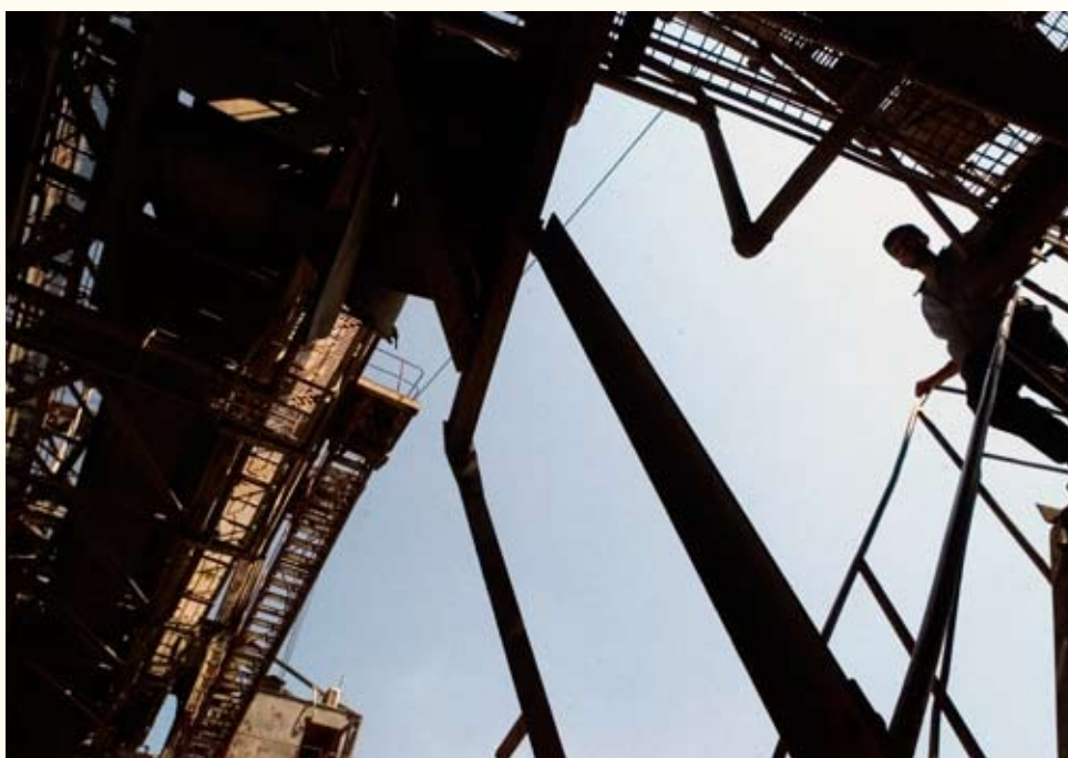
Towering tall – Coal processing facility at the Kosovo Energy Corporation power plant in Obiliq/Obilic
