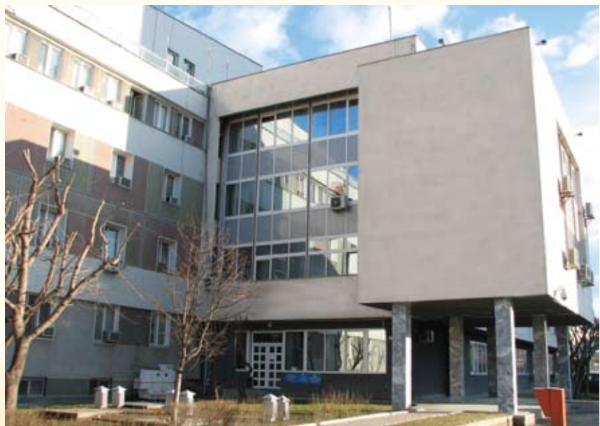
UNMIK Pillar IV premises in the Central Government Building
